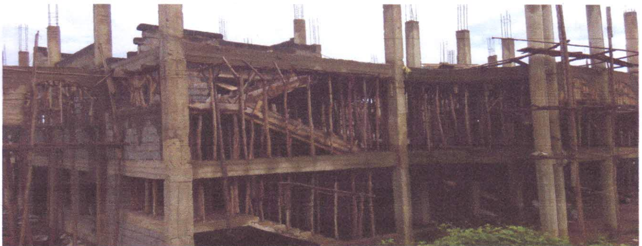
Pic 1.7.5 Kirwarwa hospital under construction
