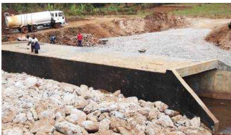
Figure 3: Rehabilitation of Mukuyu-Githambo-Kiruri Road
