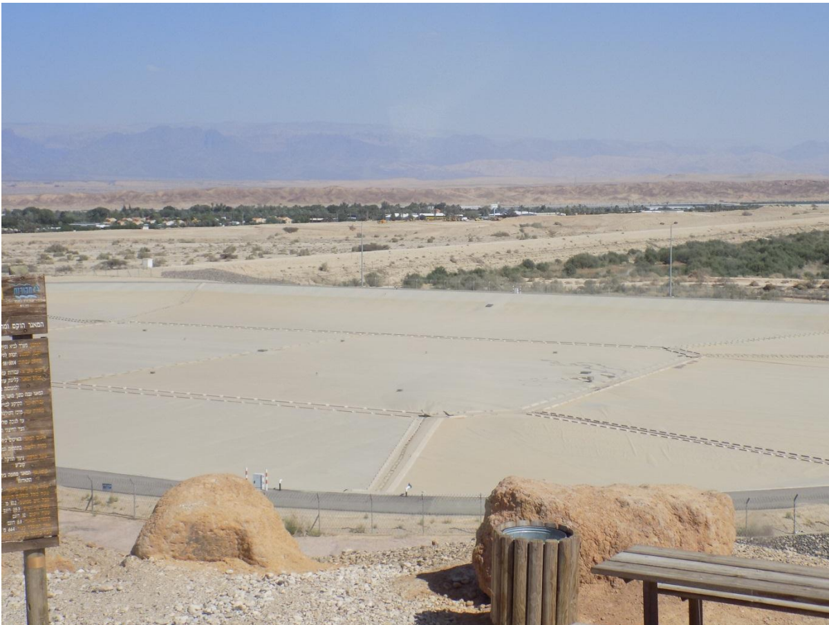
Water reservoir covered with a special polythene paper to halt evaporation and siltation.
