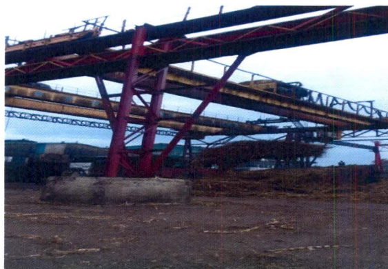
One of the machines in operation at Muboroni sugar factory
