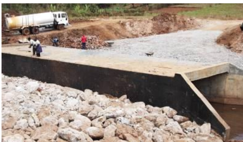
Figure 3: Rehabilitation of Mukuyu-Githambo-Kiruri Road
